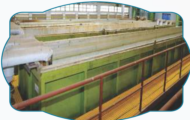
Wide Plate Pickling Tank
