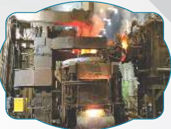
Electric Arc Furnace (EAF)
